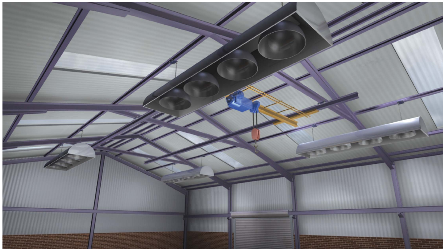
Hanging of industrial lighting systems
